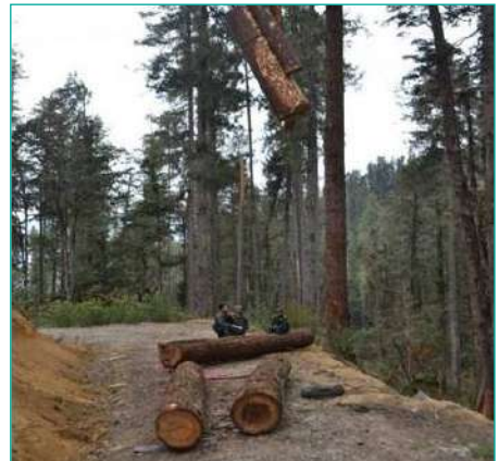
Figure 27: Skyline cable crane
