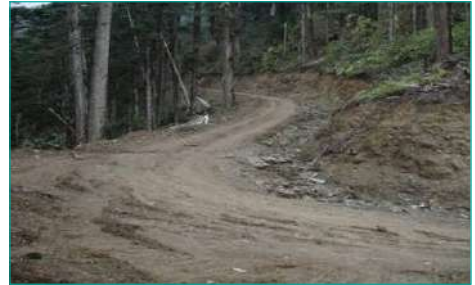
Figure 31: Forest road construction
