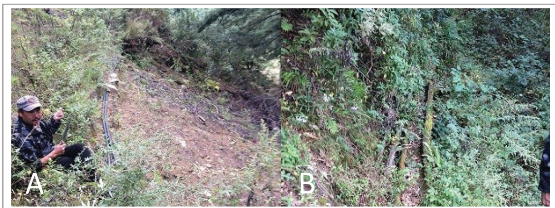
Figure 11: Landslides caused due to water loss from irrigation channel (A) and wooden irrigation channel (B), Tamzhing, April 2016.
