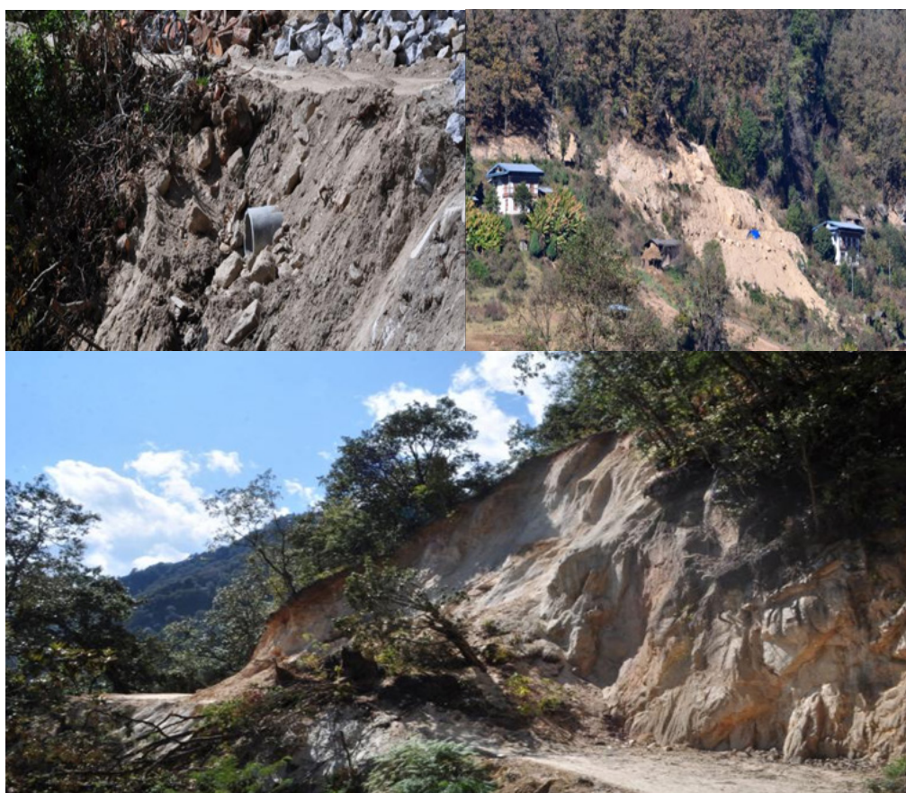
Poor quality farm roads, particularly with inadequate drainage, have led to an increase in erosion and subsequent stream sedimentation
